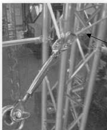
Picture 1 : Put sling around the anchorage
